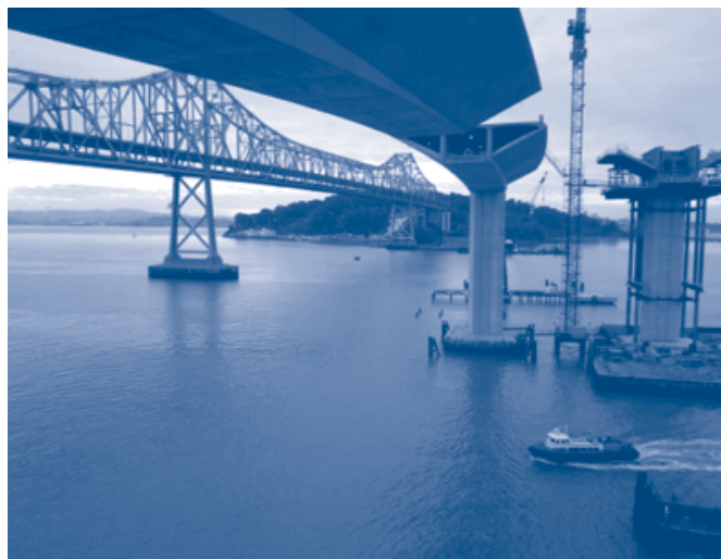
New east span under construction beside the old east span
