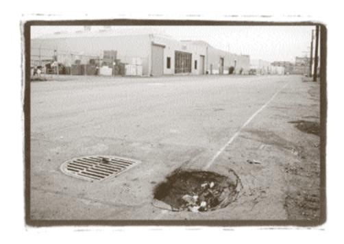
usually involves cutting a nice straight-sided hole in the pavement, perhaps digging down below the level of the current asphalt, and applying a bonding material (called a tack coat) to the sides before filling it up with new asphalt. As with new pavements, the more time spent on getting the repair right, the longer it will last. >
